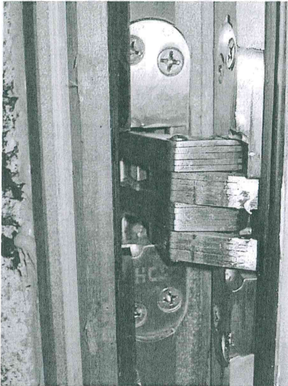
Photo 7: Fire & Smoke seal at the door leaf closing edge, fully interrupted at hinge positions
