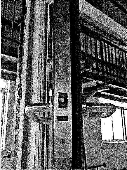
Photo 1. Door lock before the medium temperature test.
