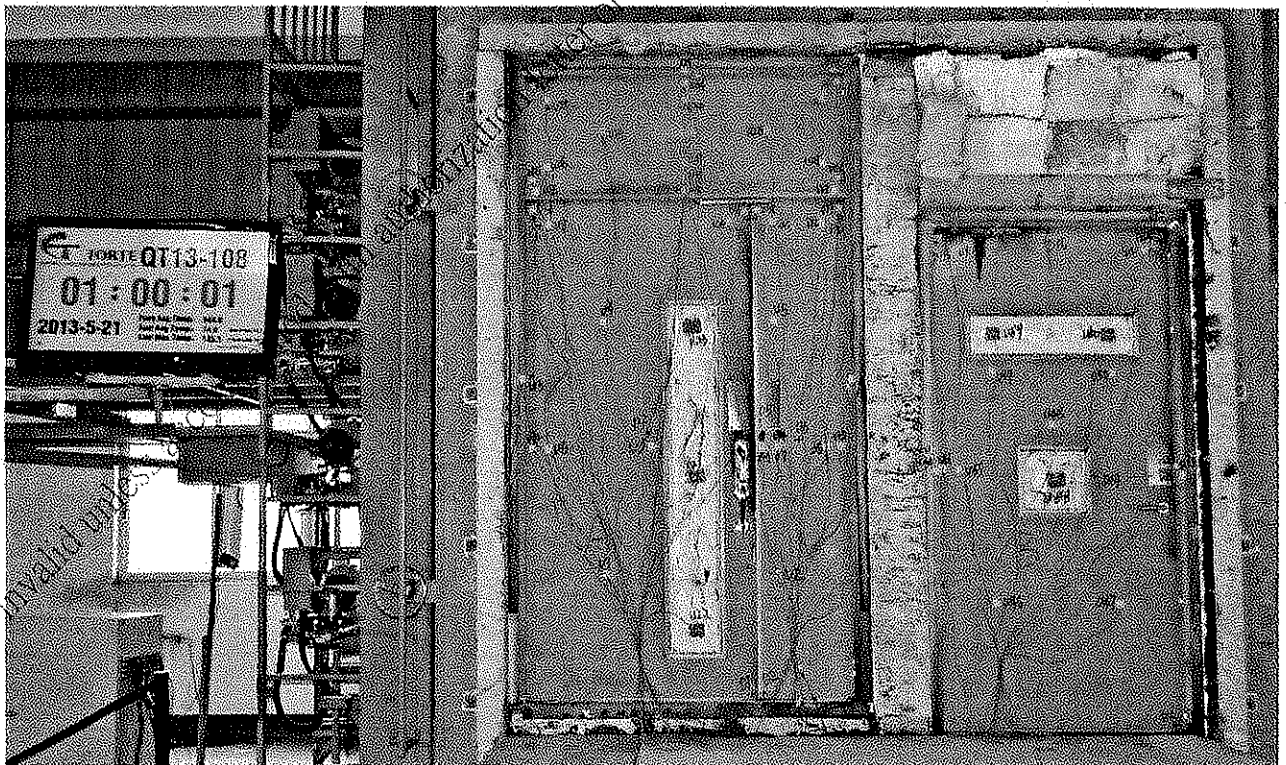
Photo 4. Unexposed surface of the specimens at 60 minute of test.
