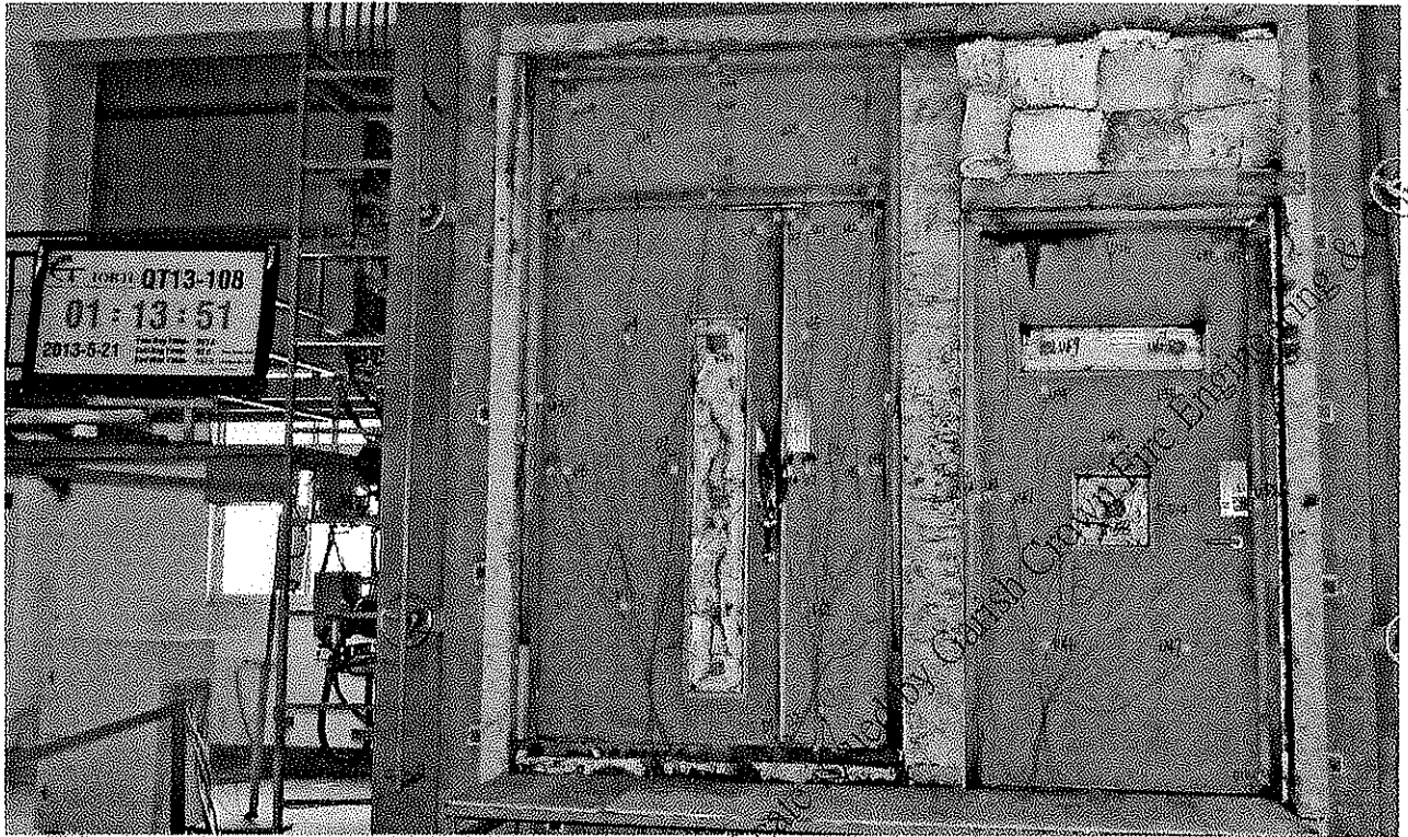
Photo 5. Unexposed surface of the specimens at 73 minute of test.
